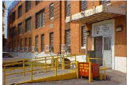
Rikers Island Hospital, which opened with the island's Penitentiary in the mid-1930s, eventually became the North Infirmary Command (NIC) above.
