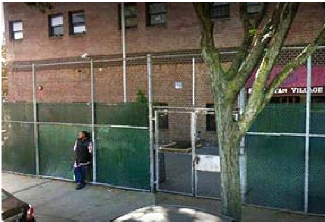
The 338 Forbell Street three-story, red-brick building, which formerly was operated as a NYC DOC women inmates jail, now serves as a shelter for homeless men.
