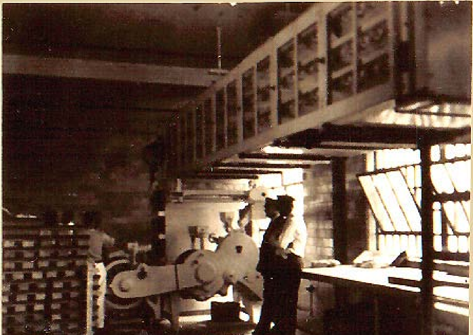
No. 7 Overhead Proofer and Moulder
